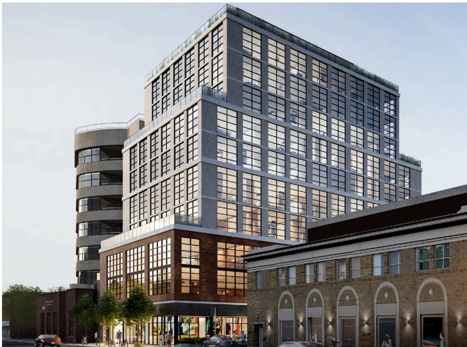
Available space at 167 Parliament will include commercial units and live/work lofts. PHOTO BY PHOTOS COURTESY OF THE DOWNING STREET GROUP AND THE SHER CORPORATION
